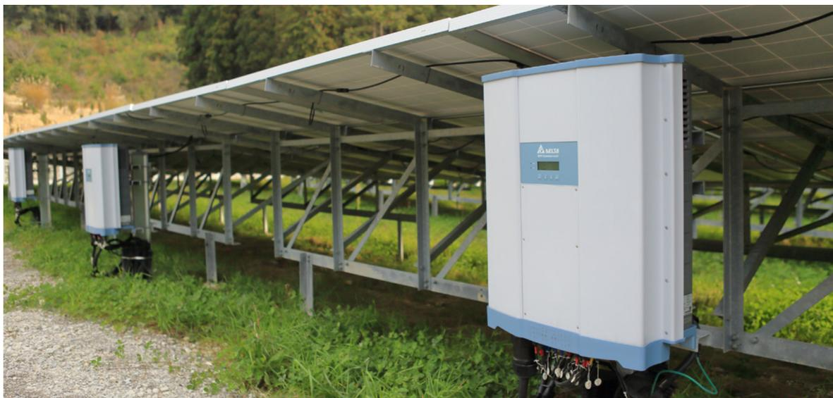
Delta's High-efficiency PV Inverters
